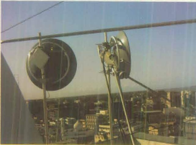
**Figure 4(a):** Two Proxim Microwave antennas very close to VSAT (partially shown on the left of the photo)
