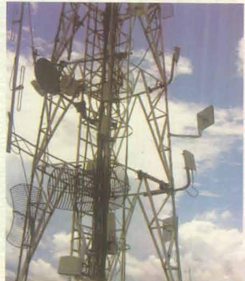
**Figure 5(b):** JM Mall Tower with Antennas. Four antennas on the right are BWA
